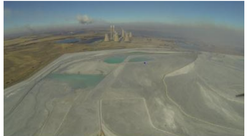
Giant ash dam next to Eskom power station. The horizon is completely obscured by smog (Photo: M Fourie)
